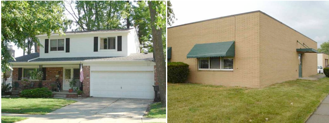
Figure TM-1 - Photographs of the two-story Welch Residence (left) and one story Marian Manor (right)
